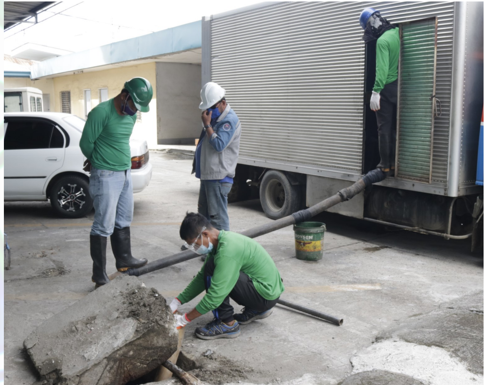
Personnel of the external service provider pumped contents of a septic tank near the PMO building 2.
